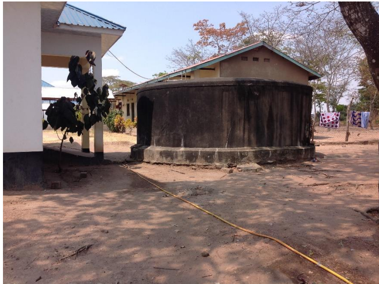
Figure 19: Rain water harvesting tank at a health centre in Bwanga Township
