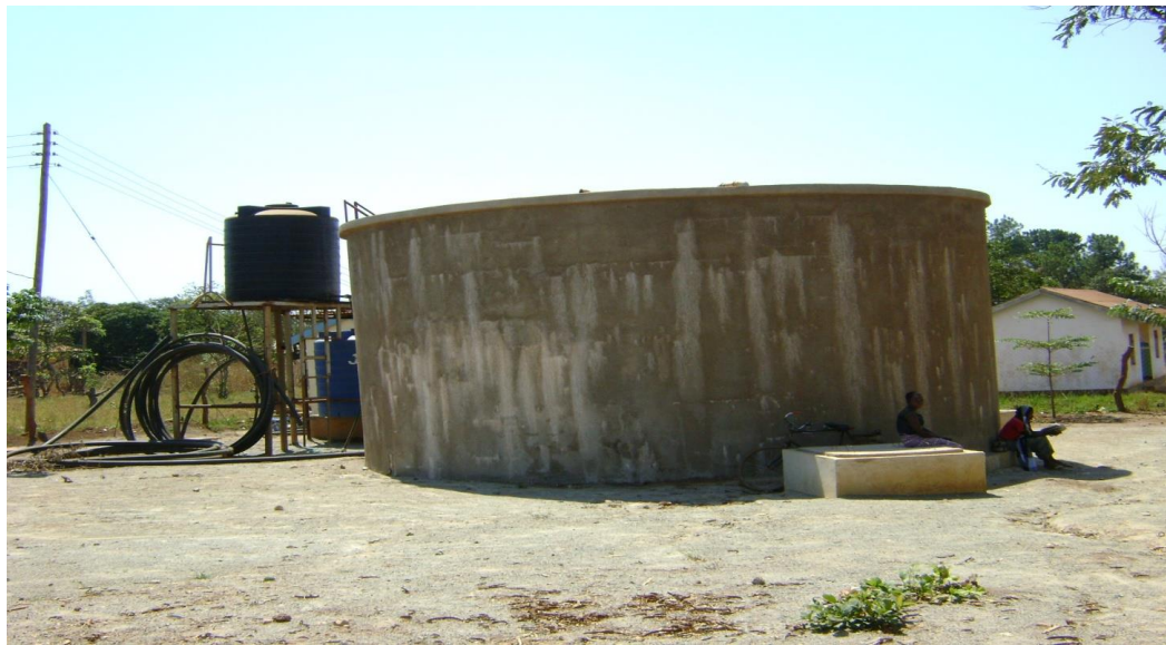
Figure 10: Water Project in Geita District Council
